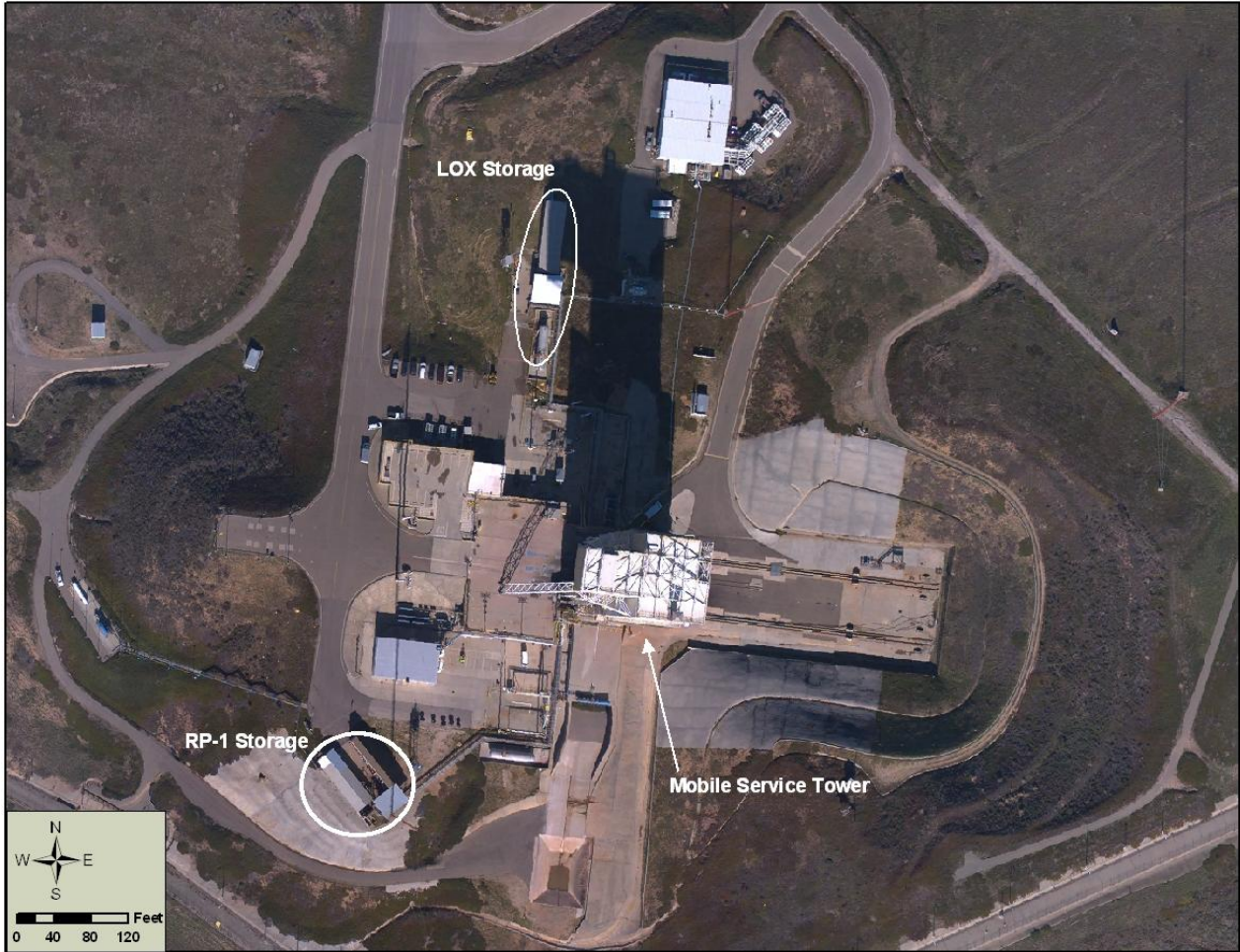
Figure 2-6. Current LOX and RP-1 storage areas at SLC-4E.
